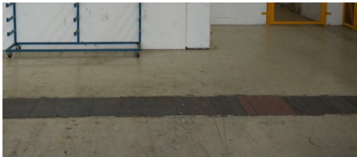
Fig. 12.8: Photograph of a typical service trench with steel covering.
