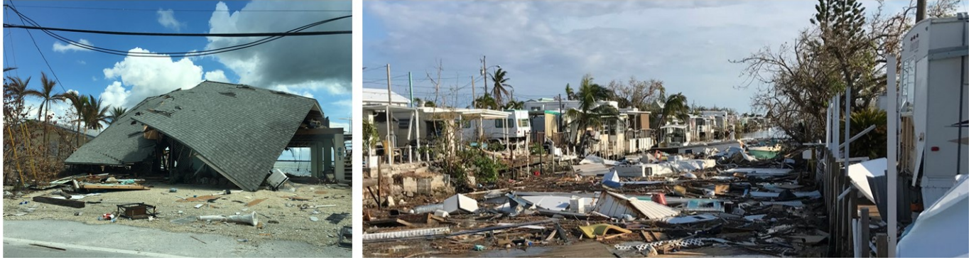
Figure 2. Photos of damage in (a) Big Pine Key: storm surge damage besides waterway (left side of building) and (b) Marathon: trailer community with house debris filling waterway
