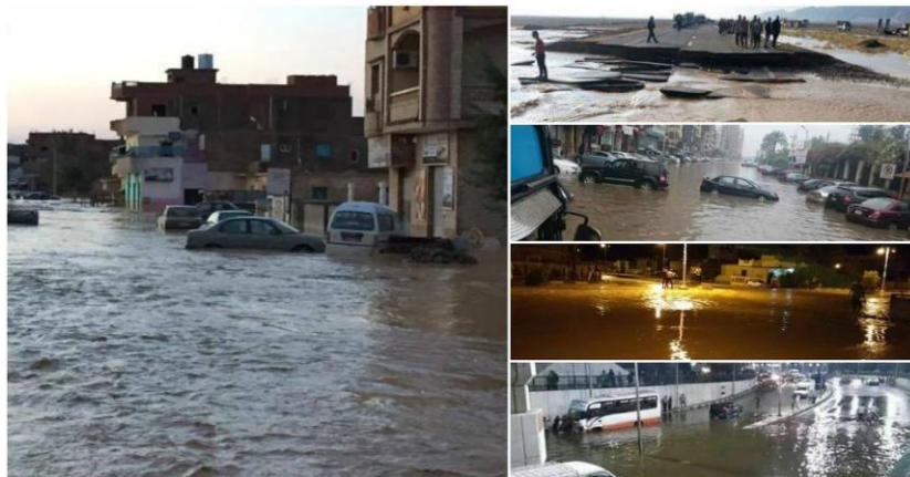
Figure 1: Damage from severe rain fall in 26 th October 2016
