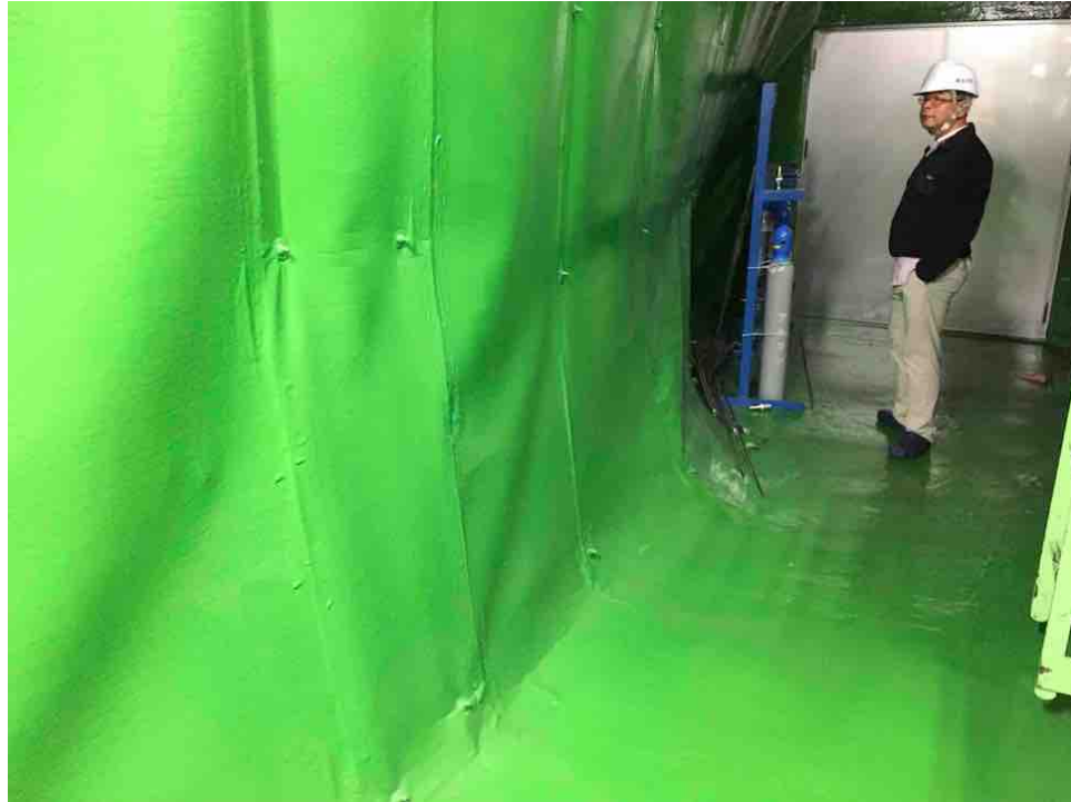
Figure 3.6: Polyethylene sheet, approx 2 mm thick, lines the rock walls, floor and ceiling, in areas where cleanliness and environment control is important. The KamLAND xenon storage and liquid scintillator purification areas are lined with this material.
