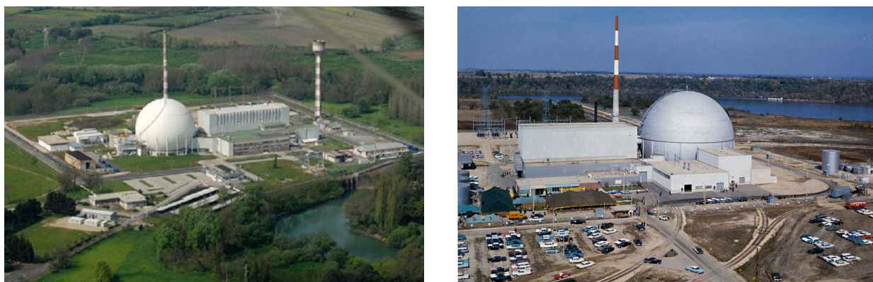
Figure 2. The Garigliano NPP – and his American twin, Dresden1 – were characterized by a containment sphere to prevent radioactivity release. In reality the containment sphere does not ensure a perfect seal, so this solution was abandoned after these two prototypes, and was replaced by more efficient containment structures.
