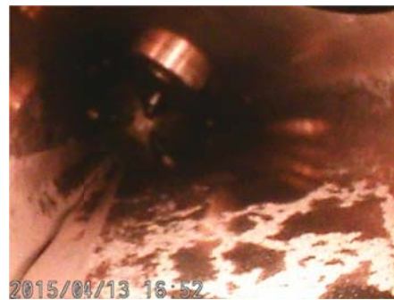
FIG. 10: RFQ surface damage status pictured from the #1 power coupler port.
