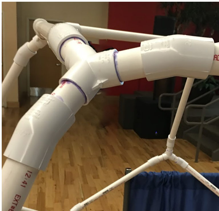
Figure 2: A close-up of the vertex joint for the dodecahedron.
