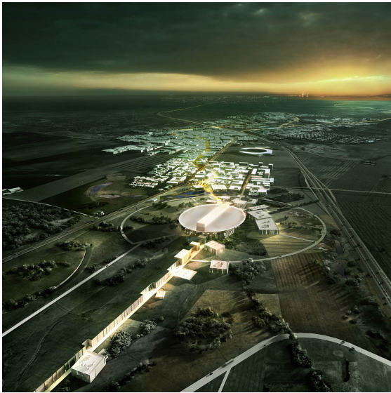
Figure 1.1: Rendering of the ESS construction project.
