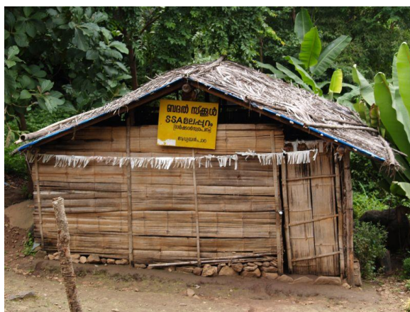
Figure 4: Tribal School at Nilambur(wikipedia entry on Tribals of Kerala)
