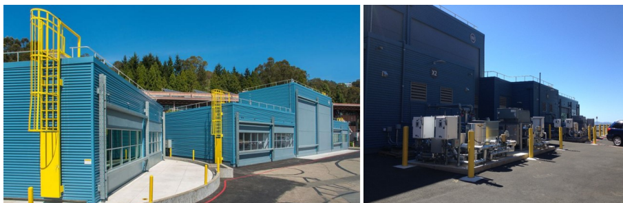
Figure 1: The Facility for Low Energy eXperiments (FLEXLAB) at LBNL.
