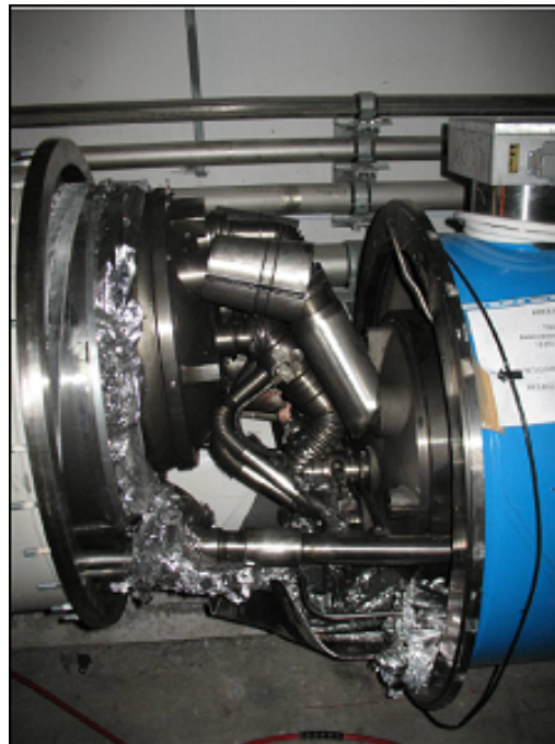
Fig. 3: Damage from the overpressure in the cryostat after the LHC accident in 2008
