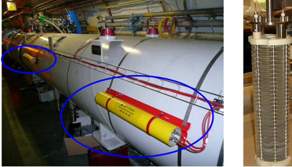
Fig. 16: Beam loss monitor at LHC
