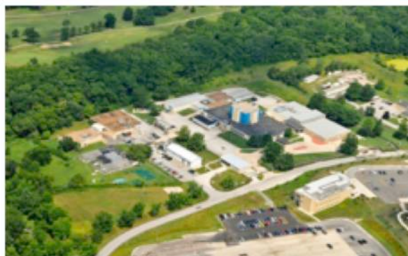
Figure 22. General layout of the MURR facilities
