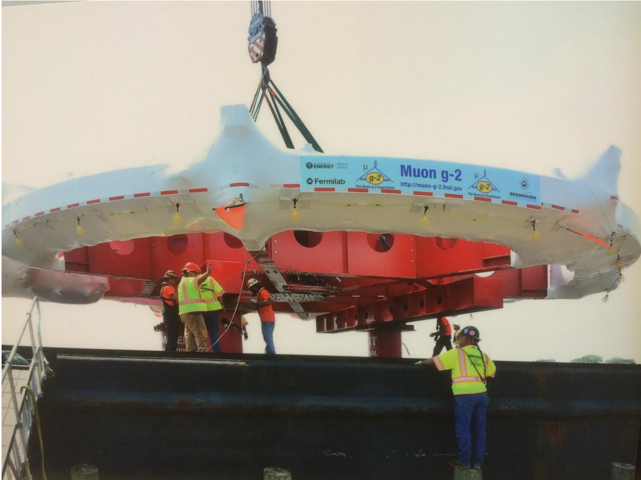
FIGURE 5. CM1 Muon g-2 solenoids ring on traveling
