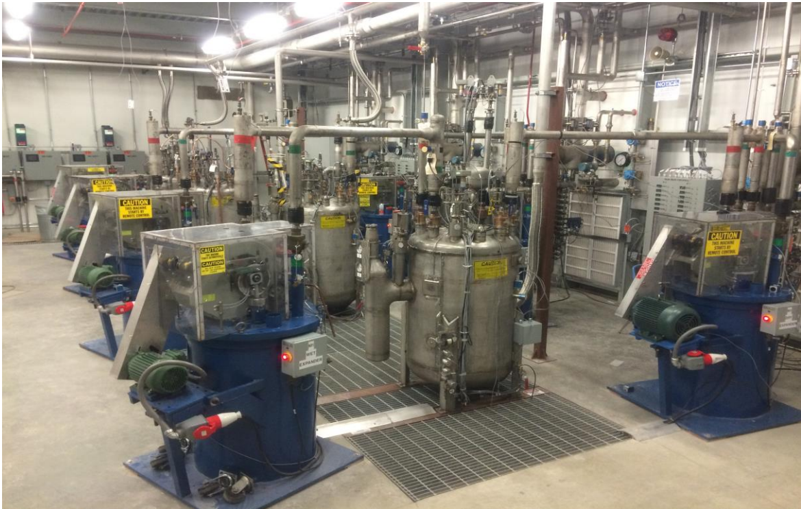
FIGURE 3. CM1 Four Tevatron style satellite refrigerators
