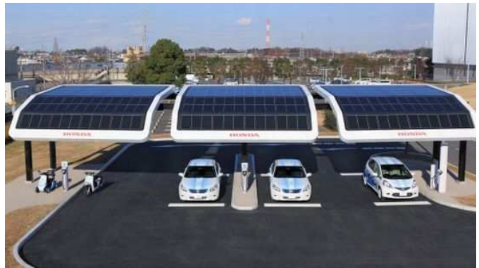
Fig. 1: An EV charging station with roof-top solar panels [38].
