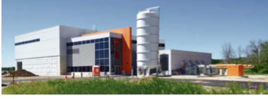
Fig. 2. The Muon Campus ( g-2 ) building captured in Summer 2014 undergoing construction.
