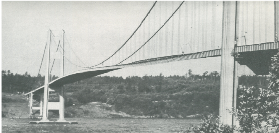
FIGURE 1. The collapsed Tacoma Narrows Bridge (1940).
