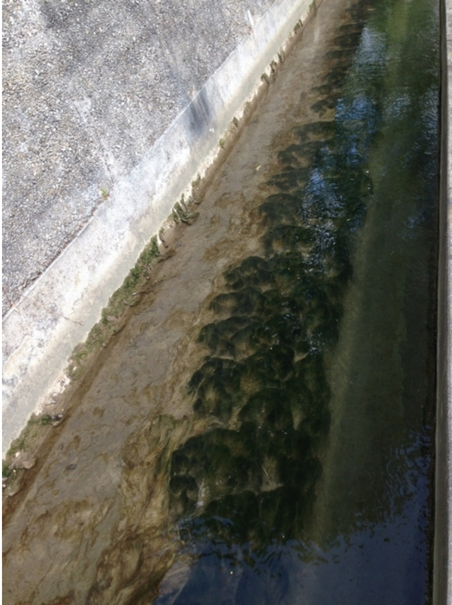
Figure 4: Concrete channel with some sediment transport and presence of longitudinal vegetation patterns; Picture credits: Paolo Perona
