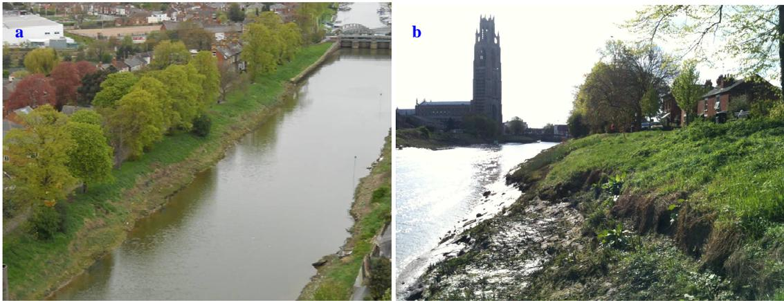
Figure 1. (a) Boston levee location at the right bank of the river Haven; (b) View of embankment with signs of toe slippage
