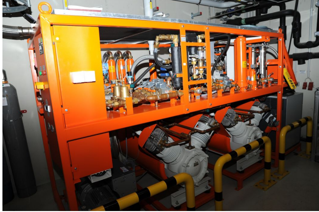
FIG. 8. Gas-handling system, including a vacuum pump and two compressors.
