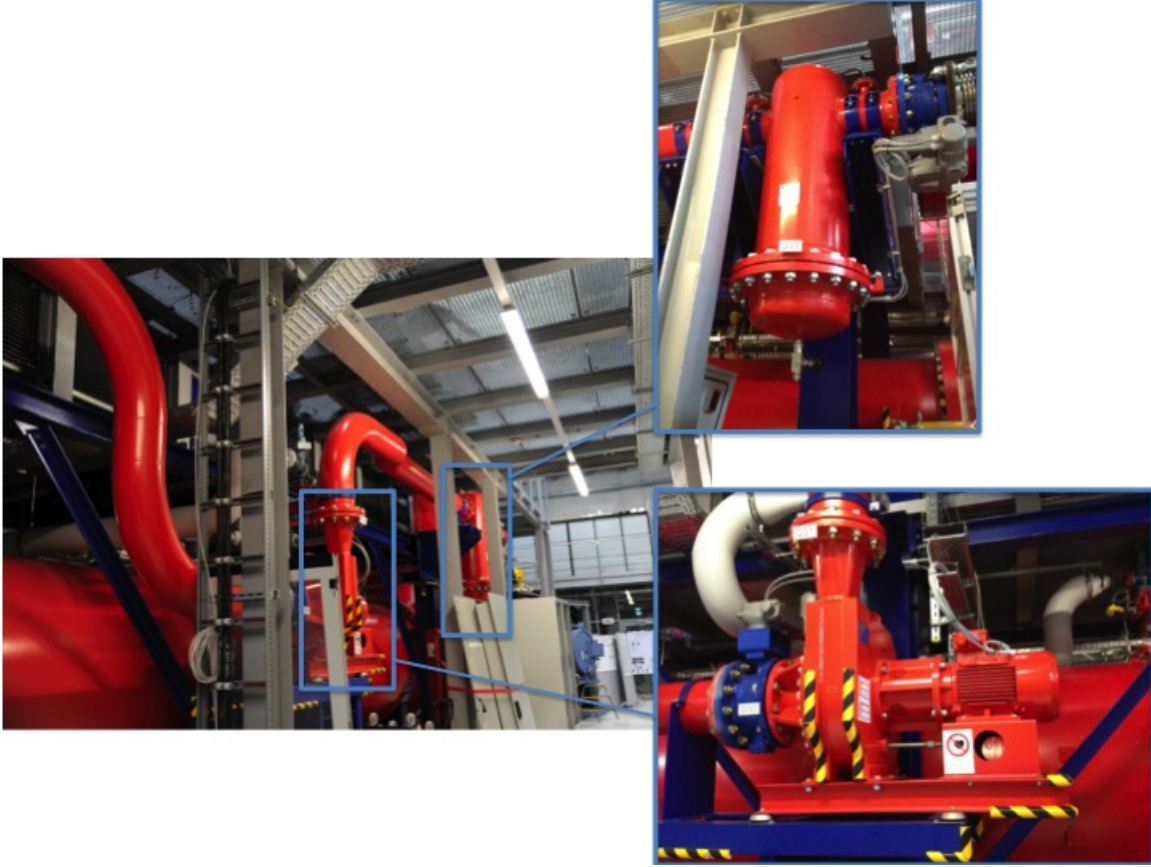
FIG. 12. Filter by-pass line with magnetically coupled pump (middle) and F9 filter cassette (end).
