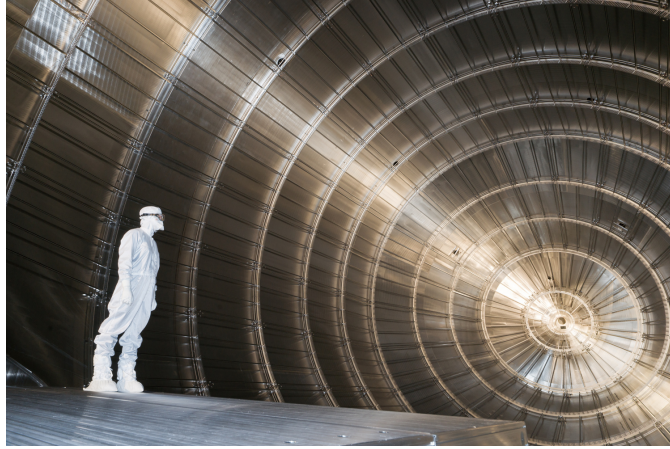
Figure 7: Wire electrode system inside the KATRIN main spectrometer during installation, photo: M. Zacher.
