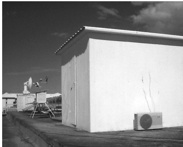
Picture 1 : Picture of the test-cell view from North-West.
