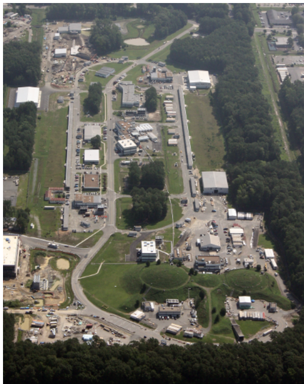
Figure 3.1 — Aerial photo of Jefferson Lab. The accelerator ring together with three round experimental halls (at the bottom) are clearly visible. The construction site for the new experimental Hall D can also be seen in the upper right corner.
