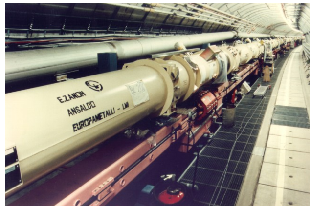
Figure 4. View of the HERA tunnel with the superconducting proton machine on top of the electron machine.
