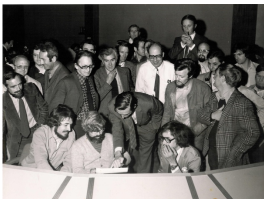
Fig. 17: SPS control room—first beams accelerated
