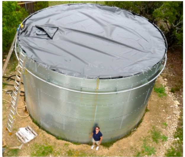
Figure 7. Test of a 7.3m diameter water tank.
