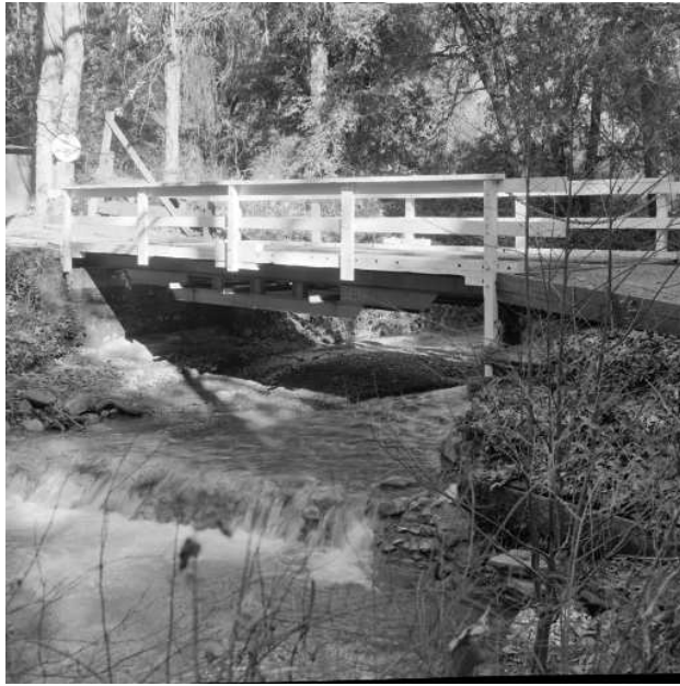
Fig. A.8. Bridge: original image
