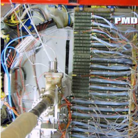
Figure 7. Photograph of the partially installed PMD in the ALICE cavern.
