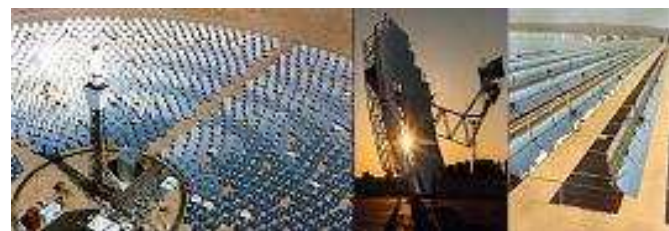
Figure 8: Concentrated solar systems. For the system in the middle photo the efficiency for producing ac electricity is ~30%.
