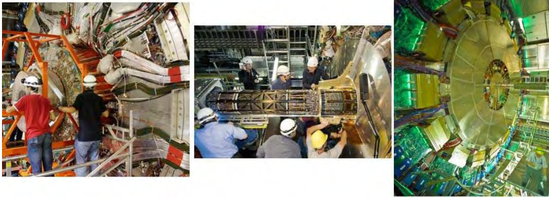
Figure 3: Left: the barrel TRT and SCT being installed in August 2006; Middle: the Pixel being inserted in June 2007; Right: the ID volume sealed with the complex end-plate with 1000 feed-throughs in April 2008.
