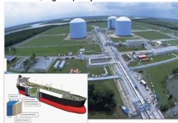
Figure 8: LNG terminal at Eba Island/ GA. The inset schematic of an LNG super tanker exhibits a hull with multiple shells. On the left a multi-layered super insulating double-hull cutout. After (DOE-NETL, 2005)
