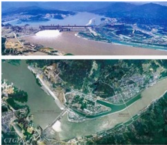
Figure 9: Two views of the Chinese Three Gorges Dam project, under construction in 2003.
