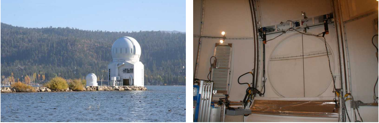
Figure 1. Left. Image of the new NST dome at BBSO. The smaller dome in the foreground houses the Earthshine and H\alpha full-disk telescopes. In this image the shutter is closed and the iris is covering the dome's 2-meter circular aperture. Right. Inside view of the closed iris and the iris drive motors. The folded windscreen is visible at the bottom of the iris.
